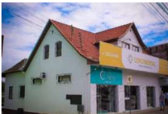
Figura 43 – Casa Comercial Huscher.
